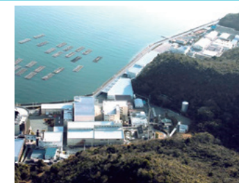
Sakoshi Plant running on renewable electricity
