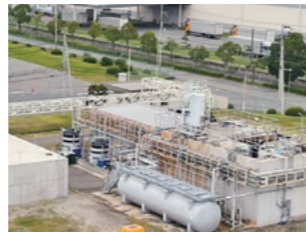
Ako Plant wastewater treatment facility
